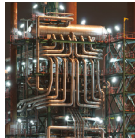
Gas compressor station
