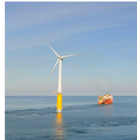
Offshore wind farm
