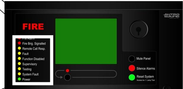
**● Fire Brig. Signalled (/ Ext. Output Activated)**
